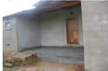
veranda at Laundry front done
