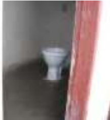
Staff toilet being done
